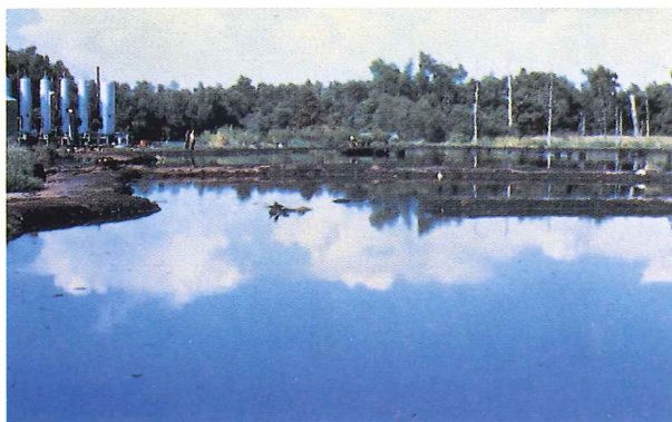
Before and after in-situ microbial degradation of heavy oil sludge over a 12-month period. OHM has 13 years experience in bioremediation.
