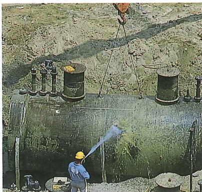
OHM performs tank removal for replacement or facility closure purposes.
