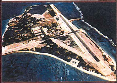
UST/AST/Pipeline Remediation, Naval Air Facility, Midway Island
