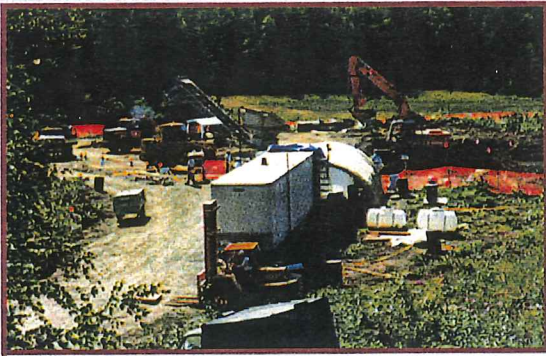
Selective Excavation/Separation/Screening of CWM Disposal Area, Fort Richardson, Alaska
