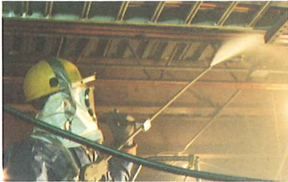
Building structure being decontaminated with high-pressure solvent spray.
