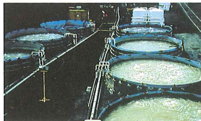
Mobile treatment systems used to treat ground water before reinjection.
