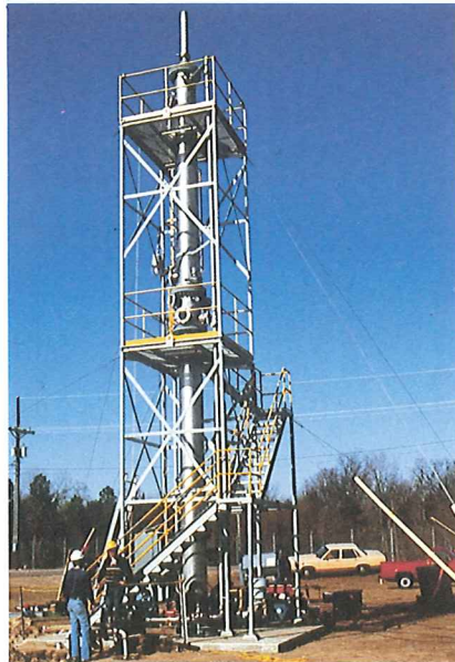
Custom designed air stripping tower removing TCE from ground water.
