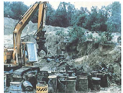
Drum grappeler lowers handling costs and increases safety of on-site personnel.
