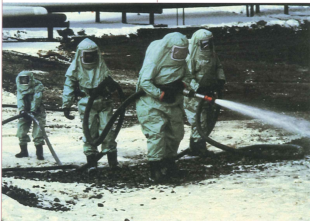
Recovery technicians oxidizing tetraethyl lead spill
