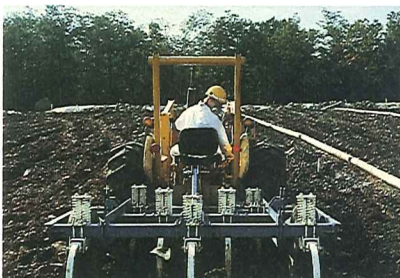
Land farming application of bacteria to treat soil contaminated with phenols
