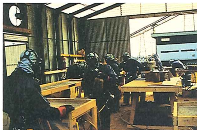
Temporary building erected for extensive lab pack operation at a hazardous waste site
