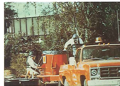
OHM designed and fabricated bomb trailer and EOD technicians removing explosives
