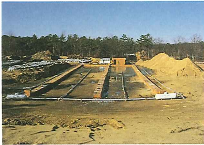
Winterized underground recovery and treatment system in place at former hazardous waste site
