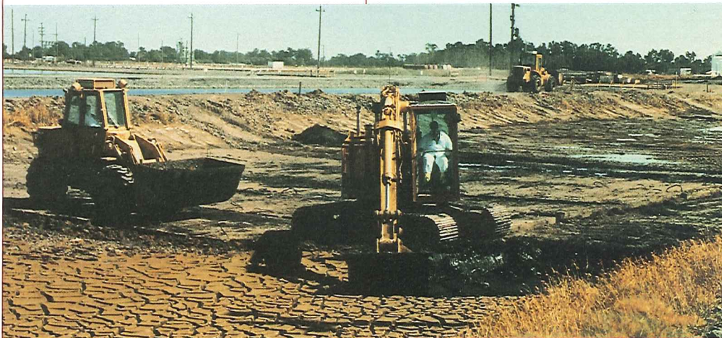
Sludge removal following lagoon treatment
