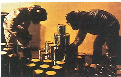
Removing material contaminated with radioactive waste
