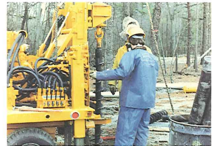
Wells are drilled for both hydrogeological investigations and groundwater recovery
