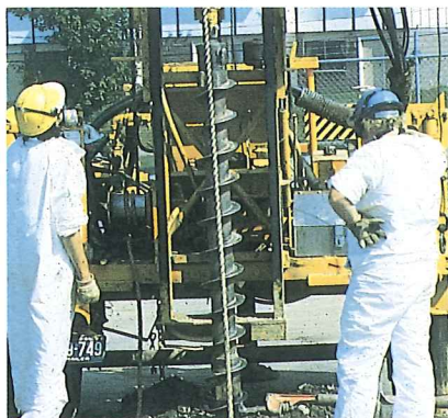
Wells are drilled for both hydrogeological investigations and ground water recovery.
