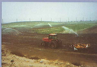
Landfarm bioremediation at a 33-acre site in Southern California in compliance with stringent state environmental quality requirements.
