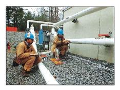
The vapor extraction system consisted of three independent well fields/vacuum recovery units. The well fields provided a channel through which vapors were pulled from the interior of the stockpile via the vacuum pumps and transported to the regenerative thermal oxidizer for destruction.
