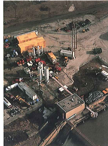
Design, engineering, fabrication, installation and operation of 5-million-gallon-per-day water treatment system completed in nine days
