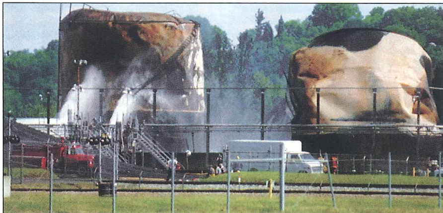
Explosion-damaged Shell plant in Ohio is typical of OHM's emergency cleanup response work.
