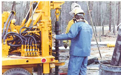
Wells are drilled for both hydrogeological investigations and ground water recovery
