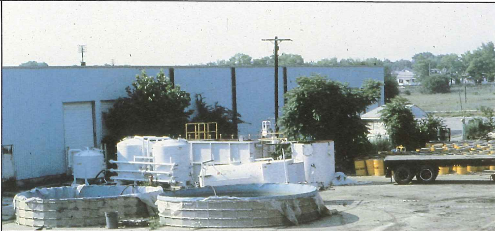
Diagram and photo show typical on-site system for treatment of contaminants: (1) vacuum receiver (2) transfer station (3) clarifier (4) mixed media pre-filter (5) carbon filter (6) 12,000 gal. pool (7) 22gpm HYDRO-LASER.
