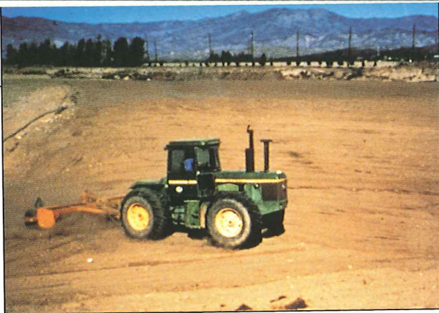
FIGURE 2. Tilling with agriculture-type equipment enhances soil aeration and speeds up land treatment
