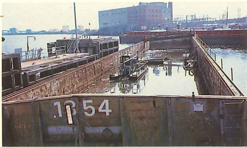
Hopper barges for storage of 400,000 gallons of sediment awaiting processing
