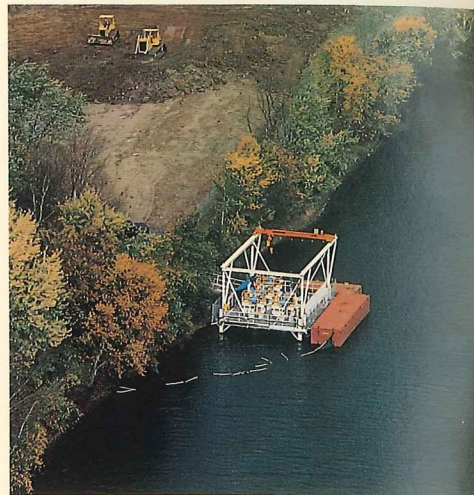
Three-month demonstration project to determine feasibility of bioremediation of PCB-contaminated river sediments
