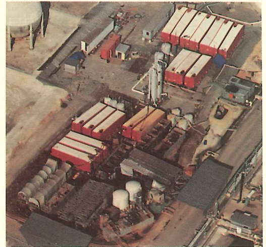
Five-month project completed without disrupting manufacturing plant or shipping operations
