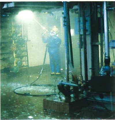
Above: Sampling and Overpacking of Unknown Chemicals Upper Left: Major Remediation Project Site Left: Hydroblasting PCB-Contaminated Facility
