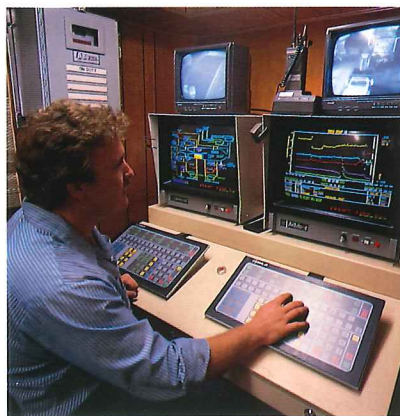
Above: Mobile Incinerator at NPL Site Upper Left: High Efficiency Plate and Frame Filter Press Left: Mobile Incinerator Control Center
